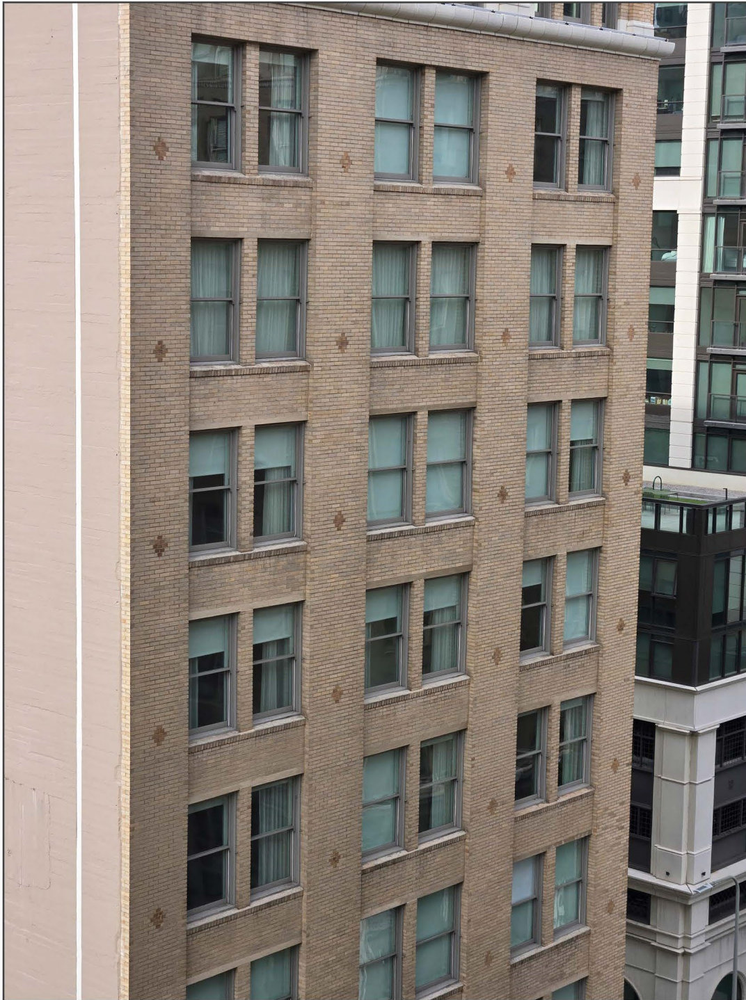
4. View west of eastern elevation building shaft from rooftop of 800 South Spring Street.
