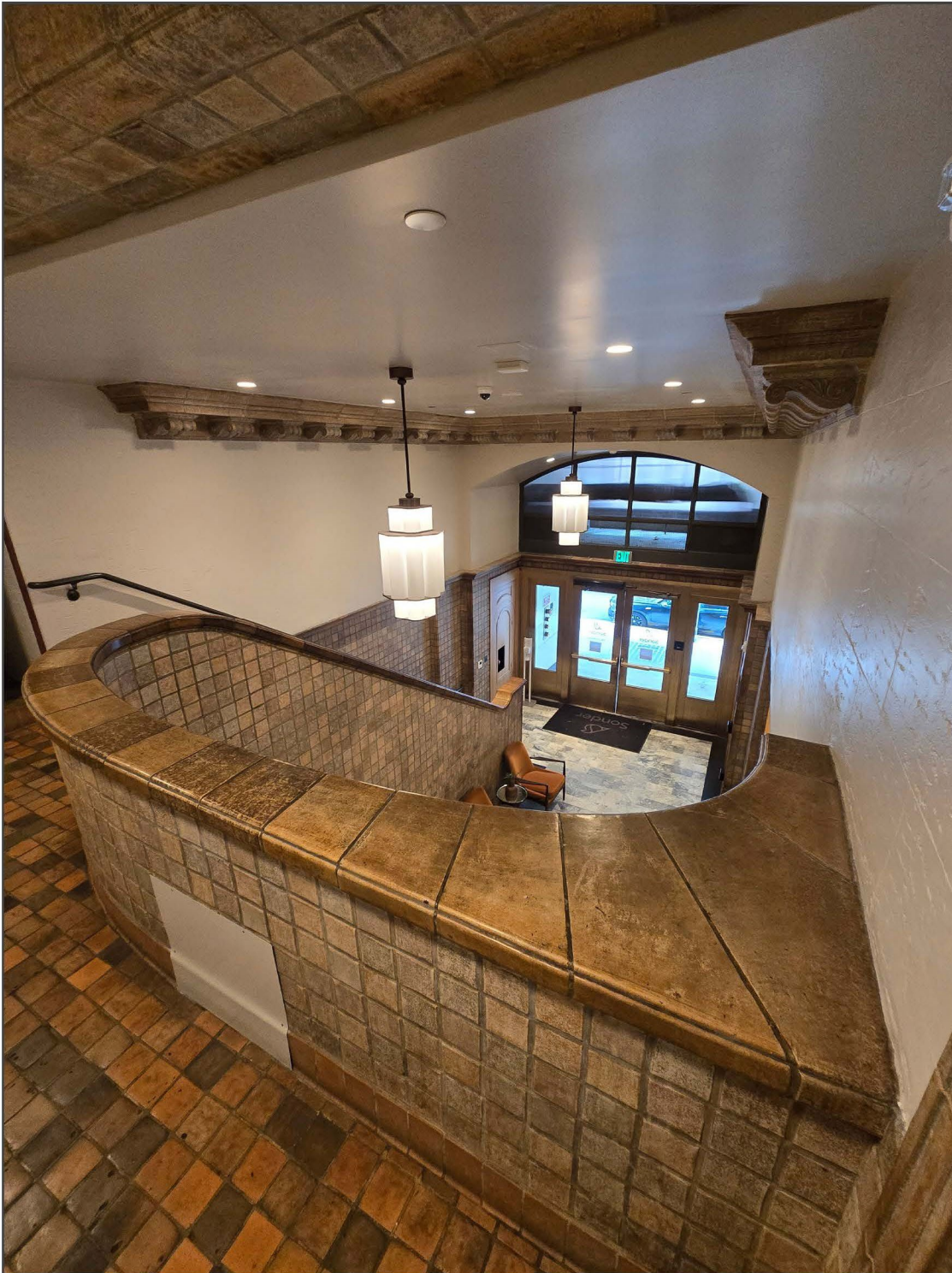
13. Mezzanine: View northwest of lobby illustrating balustrade, coping, and cornice.
