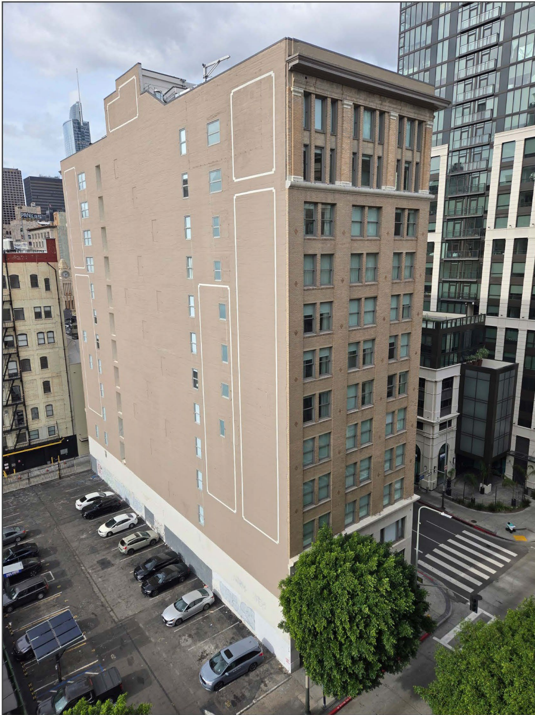
3. View northwest of east and south elevations from rooftop of 800 South Spring Street.
