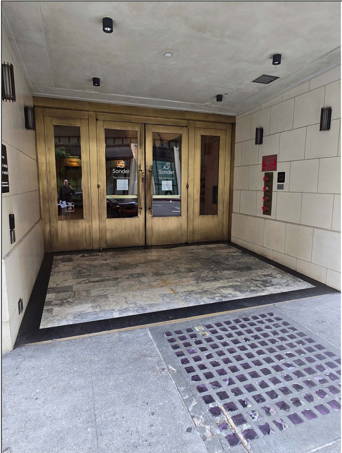
7. View south of recessed foyer and lobby entrance from sidewalk along West 8th Street.
