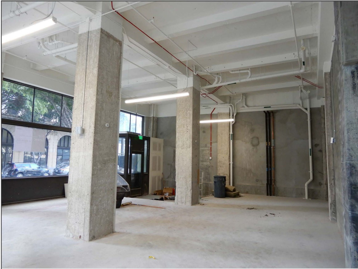
16. Retail 3: View southeast within retail toward South Spring Street entrance.
