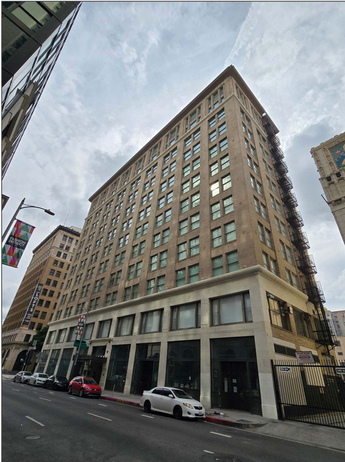
2. View southeast of primary (north) and west elevations from West 8th Street.
