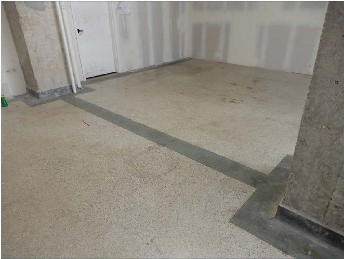
14. Retail 1: View southwest of retail space including concrete columns and terrazzo floor.
