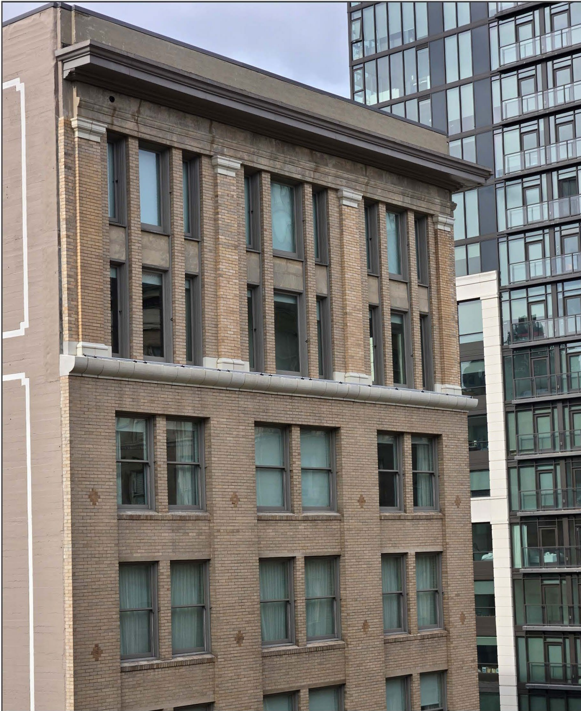
5. View west of eastern elevation building capital from rooftop of 800 South Spring Street.
