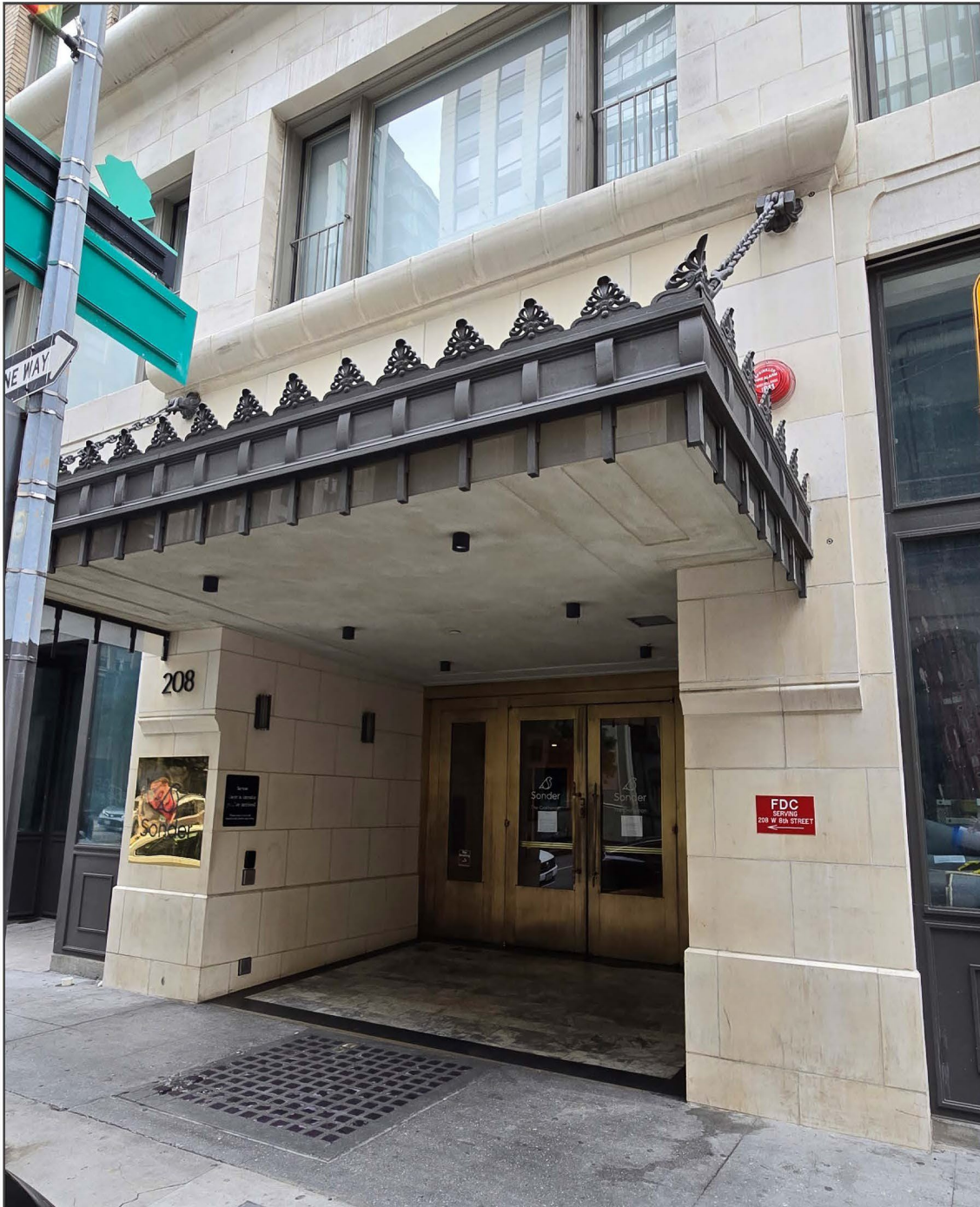
6. View southeast of canopied main entrance from sidewalk along West 8th Street.
