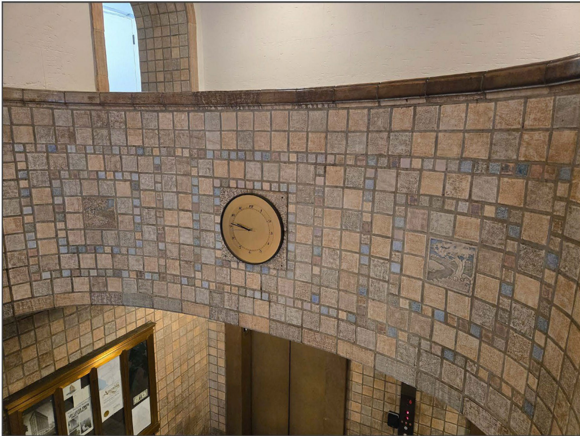
12. Mezzanine: View southwest from the stairs of feature tiles and clock that comprise the mezzanine balustrade.
